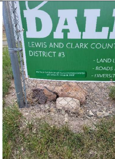
N Montana Ave near West Valley VFD
